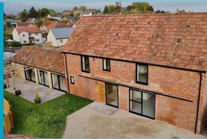
Refurbishment - Grade II
